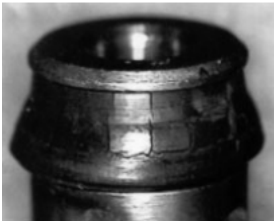
Photo 2 Cracking of check valve seal
